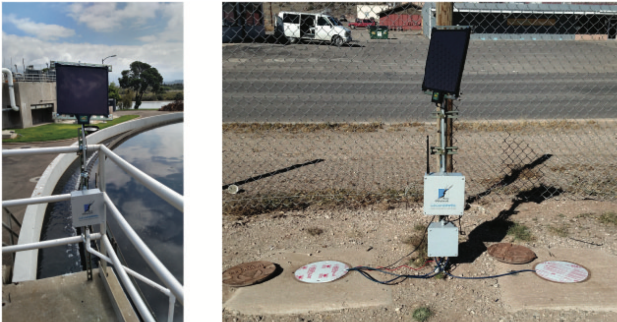
Figure 1: Photographs of field deployments: Goleta wastewater treatment and Grants Superfund Site
